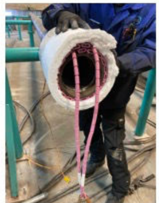
4. WRAP PADS WITH INSULATION
