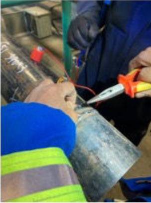
5. CREATE A THERMOCOUPLE INSIDE THE HEAT TREATMENT AREA
