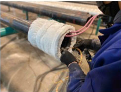
5. CREATE A THERMOCOUPLE INSIDE THE HEAT TREATMENT AREA
