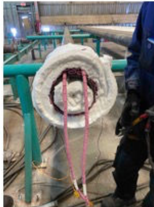
6. INSULATE INSIDE OF THE PIPE
